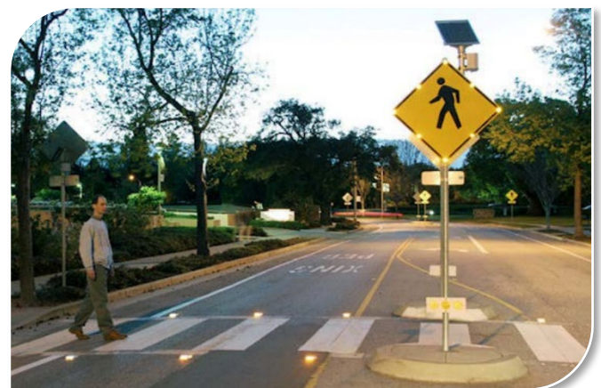
Figure 91. Solar-powered pedestrian crossing system.
