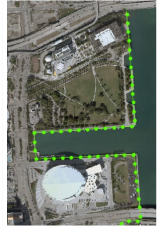
Figure 2. Paved path from Bayside to Kesaya Center
