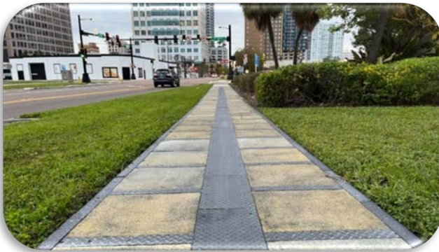
Figure 81. Solar panel technology installed on sidewalk in Tampa, Florida.
