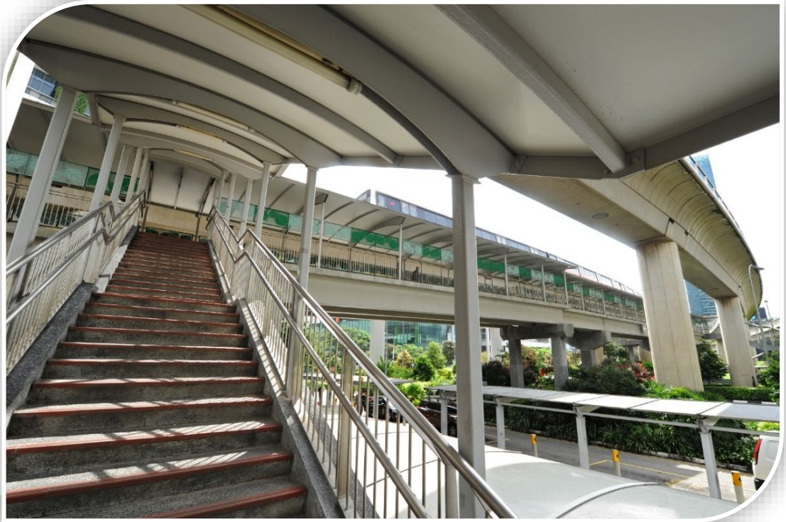
Figure 9. Sheltered skyway near a transit station in Singapore.
