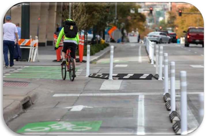
Figure 101. Example of Denver Wedge installation.
